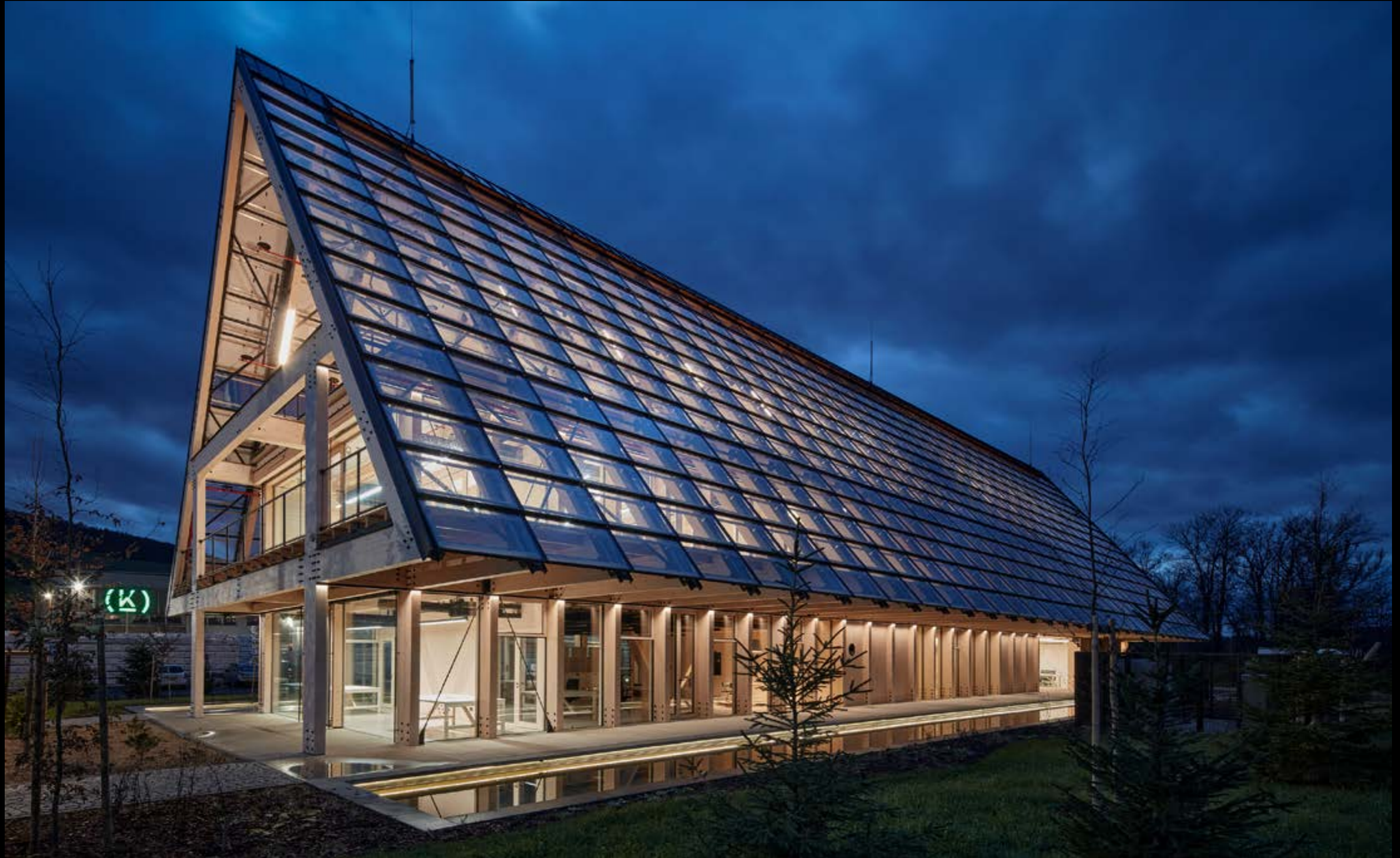
A clever and clear design: While on the north side of the building the wooden structure is exclusively covered with glass panels, more than half of the south side is covered with photovoltaic modules (photo: BoysPlayNice)
